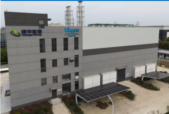
Microgrid Demonstration Project In Jiangsu Province
